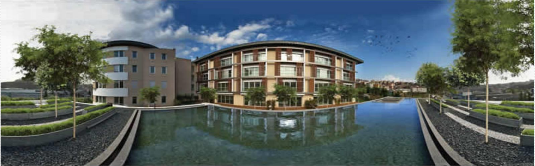
Bay İnşaat Hill Park Suite İstinye ( 2 Blok 91 Daire – Sosyal Alan )
